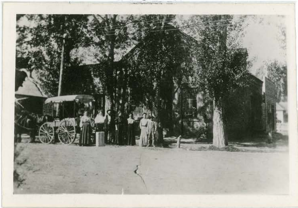
Remodeled Wellsville Cooperative Store Figure 4
